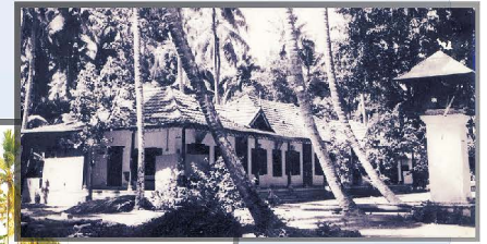
Maliampurackal house at Pulincunoo village
